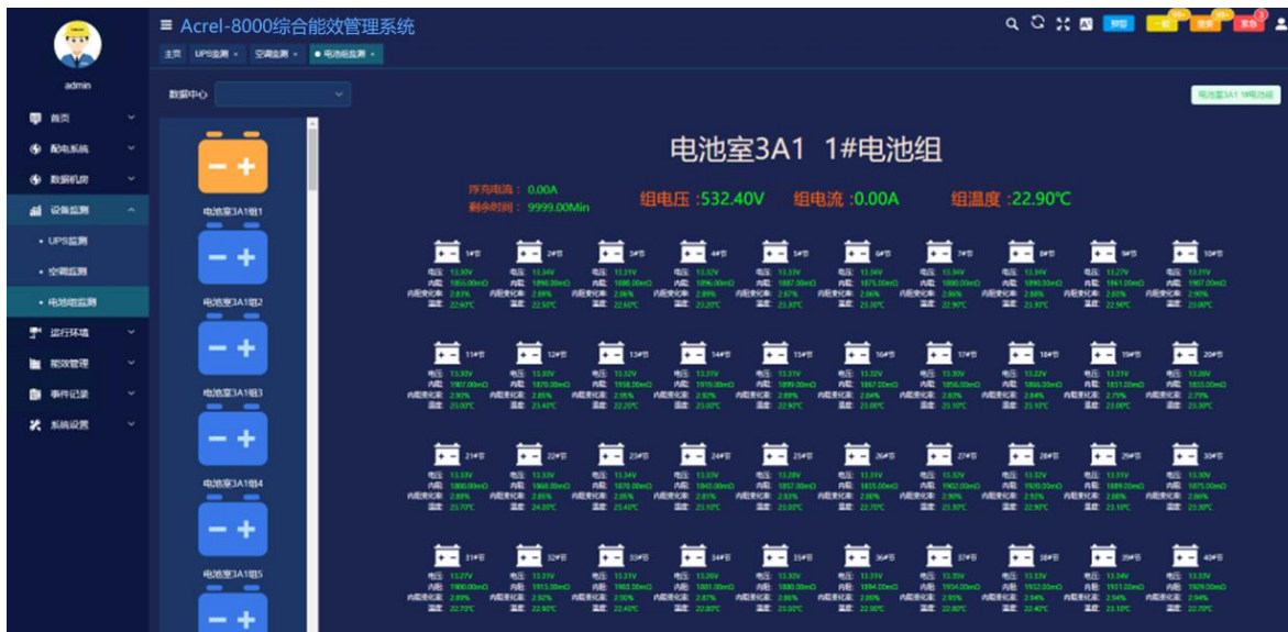
Monitor battery pack voltage, current, floating current, pack temperature. Voltage, internal resistance, temperature of a single cell.
